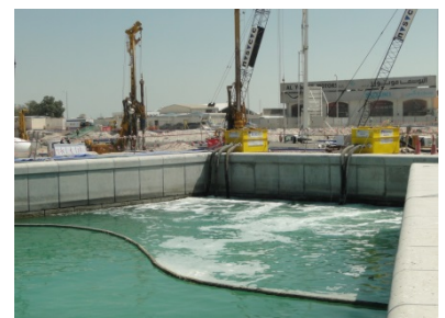
Silt curtain at dewatering discharge point.
