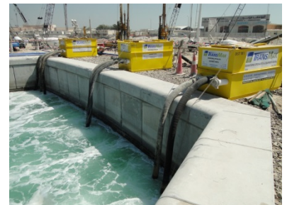
Settling tanks discharging into the sea.
